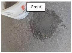
Mix 2 ounces A with 2 Ounces B with 4 ounces Part C colored the same measurements as patch. grout surface of repair.
