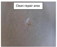
Chip out loose or foreign debris and vacuum sample repair area on floor.
