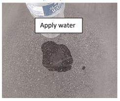
Grind flush with concrete and apply clean water to repair surface. Let completely dry and Polish to #400.
