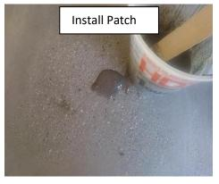
Mix resin and part C. Overfill repair 1/8". Let cure 30-50 minutes and grind flush with concrete.
