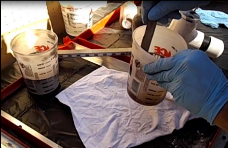
5. Mix A and B quickly to streak free.
