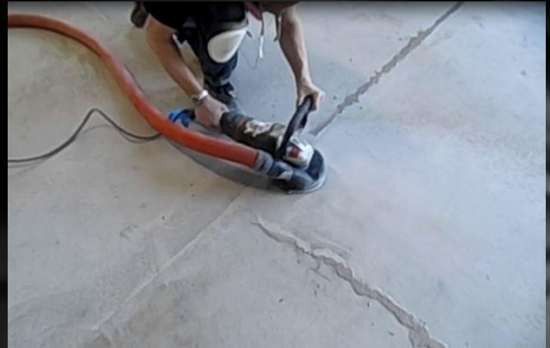
2. Grind cured patch flush with concrete.
