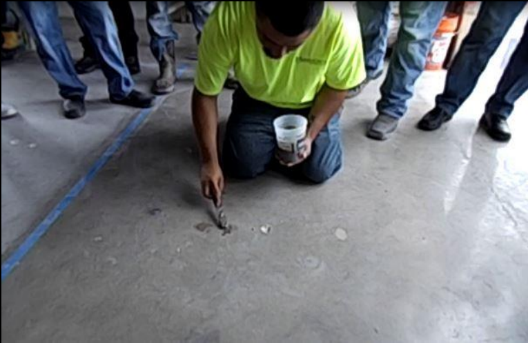
1. Install mix into cleaned repair, over fill.
