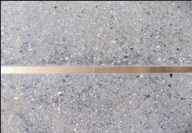
Joint re-build Polyurea, brass and zinc.
