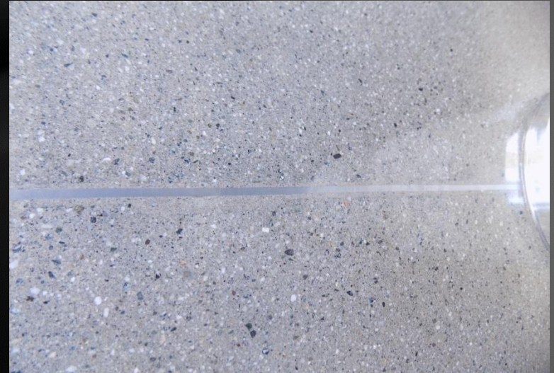
Joint re-build Polyurea, brass and zinc.
