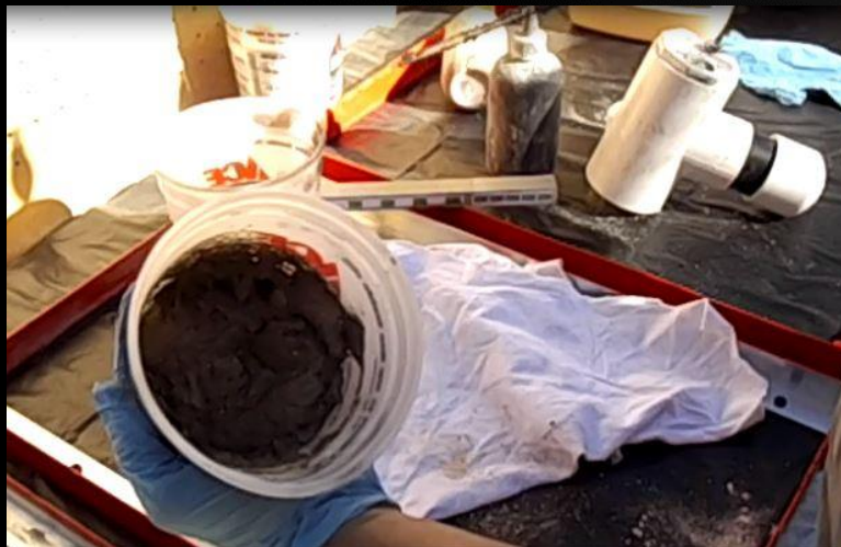
7. Mix remainder of part C/sand "peanut butter."
