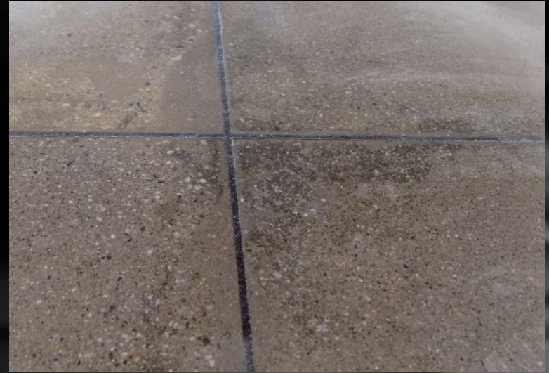
Joint re-build Polyurea, brass and zinc.
