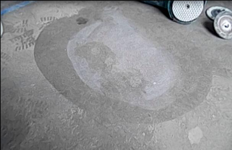
3. Topically add water to top of patch. Let soak in 10 minutes and dry completely.
